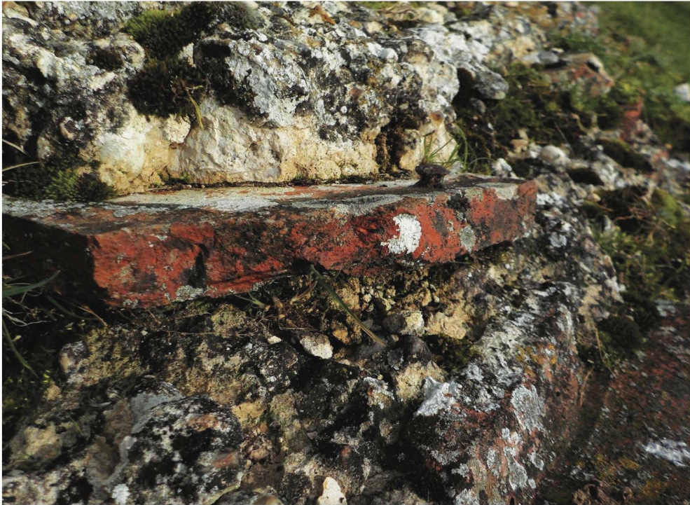
Fig. 5 A tile, with nail in situ, reused in a tile course of the western wall. (Photo by M. Davies.)
